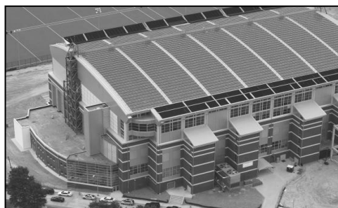
Fig. 1. Aquatic Center Roof-Top PV Array
